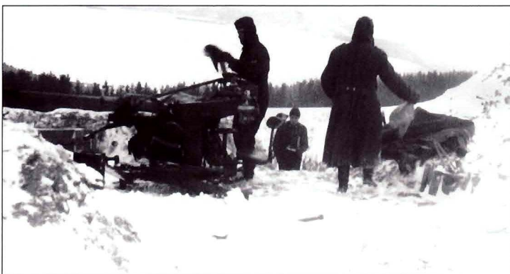
A Luftwaffe crew services its 2cm Flak 30 set-up in a frontline position. Though normally covered by a canvas tarp, it had to be checked a couple times a day to ensure there was no ice build-up in the firing mechanism and operating controls. It also had to be re-oiled. Note the gun shield has been removed.
