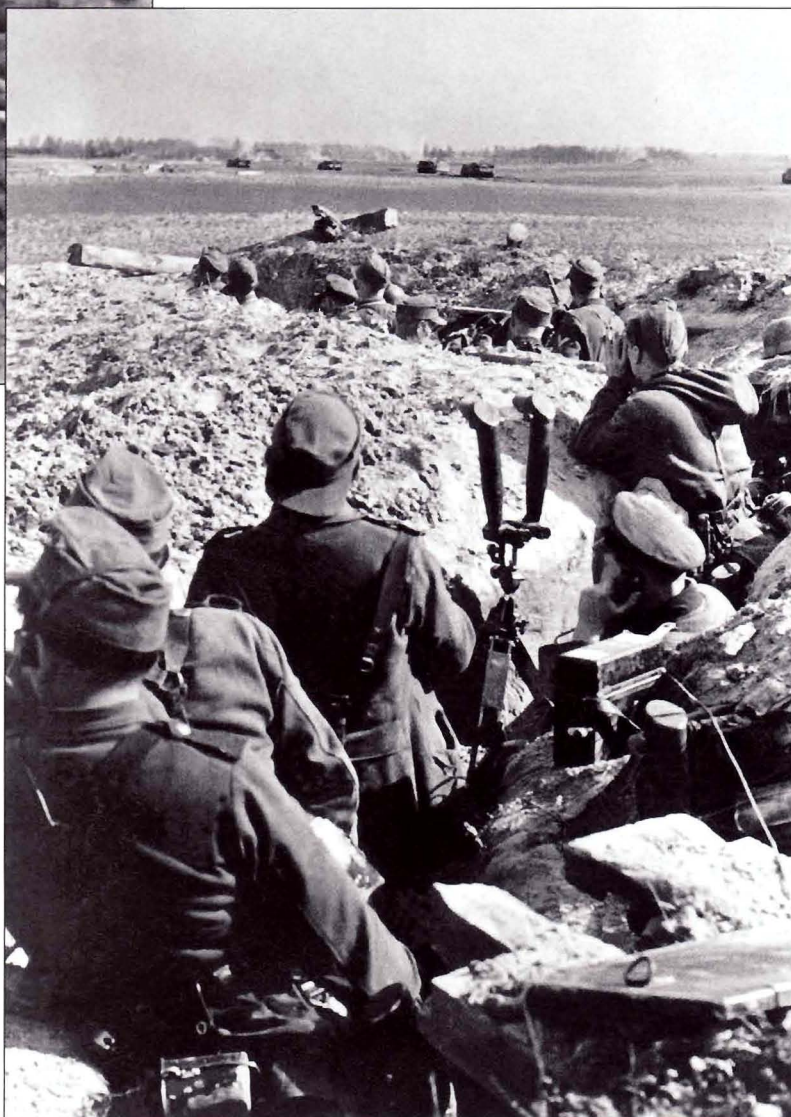
This artillery battery observation post has obviously been co-located in an infantry trench. Observation posts were not normally so crowded. A Feldfernsprecher 33 in its Bakelite case can be seen to the right of the Sf.14Z Scherenfernrohr. It appears that an assault is being launched as a column of assault guns advance. In the original photograph there appears to be faint puffs of smoke on the distant treeline.
