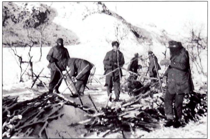
Gebirgstruppen wearing the sage green windbreaker for mountain troops (Windjacke für Gebirgstruppen) assemble Spanish riders (spanische Reiter) barbed wire-wrapped portable anti-personnel obstacles. These are also known as knife rests or chevaux de frise. These particular knife rests appear rather flimsy as most were built of thick logs. Once emplaced and drifted over with snow they were quite difficult to pass through, especially if positioned among bushes also covered by snowdrift. Winter 1943/44.
