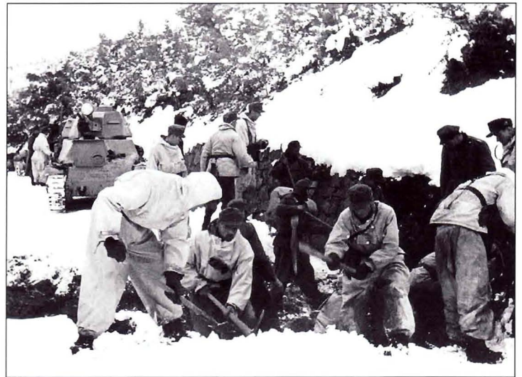
Pioneer troops hack out a hasty antitank ditch as a temporary roadblock during the seemingly endless retreat. The easiest way to do this in a hard- or packed-surface road in frozen ground was to use demolition charges, at least to provide starter holes. However, in this instance it does not appear that demolitions were available or there would be rocks and dirt clods scattered all about.
