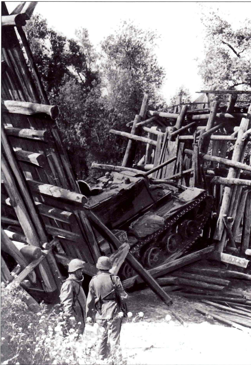
German troops examine a timber bridge unable to bear the weight of a Soviet KV-1 tank. The crew in all probability survived the collapse. The soldier to the right is armed with a 9mm MP40 machine pistol and a pistol, probably a 9mm Walther P38.
