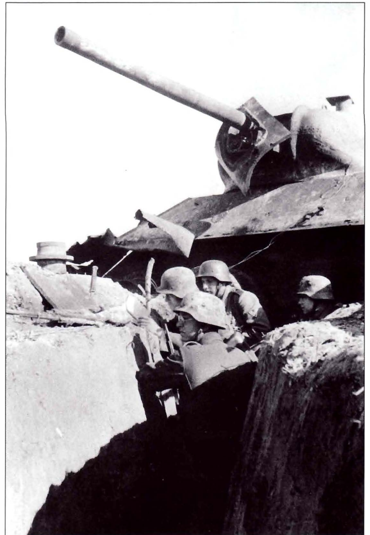
A bunker has been built beneath a T-34/85 tank to provide effective protection from artillery. One disadvantage was that it provided the enemy with an easily identifiable landmark for directing fire at and pin-pointing the trench's location. Nevertheless, damaged tanks provided a rapidly constructed bunker with significant overhead cover. A severely damaged rifle, probably uncovered when the trench was dug, lies on the left lip of the trench.
